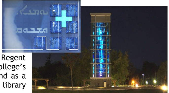
The Regent College wind tower by night - a beacon for the surrounding park
