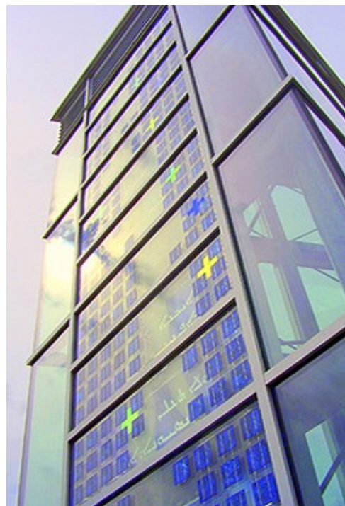
The stained glass with PV is the central element of the Regent College wind tower at the University of British Columbia/ Vancouver
