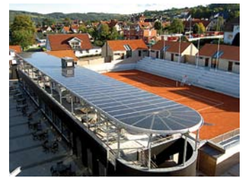
Some 80 kWp is installed at the Båstad Tennis arena, home of the Swedish Open tournament. [PHOTO: GLACELL/SHARP]
