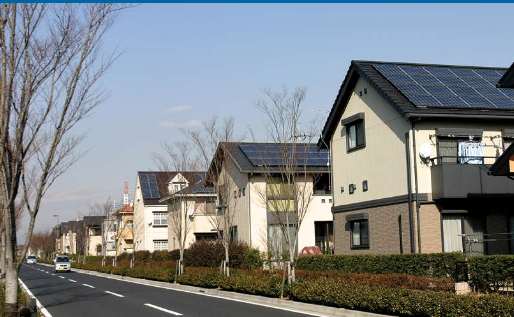
Pal Town Jyosai-no-Mori in Ota City, Gunma Prefecture is a prime example of an intensive PV integration into newbuild housing. The development totals over 2,1 MW across 553 houses.
