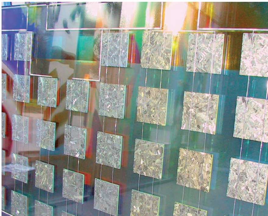
Students will get a firsthand look at how solar cells provide power through this installation of art glass in the entryway stairwell of Grass Valley Elementary School in Portland, Ore. Photo courtesy of Sarah Hall Studio.
