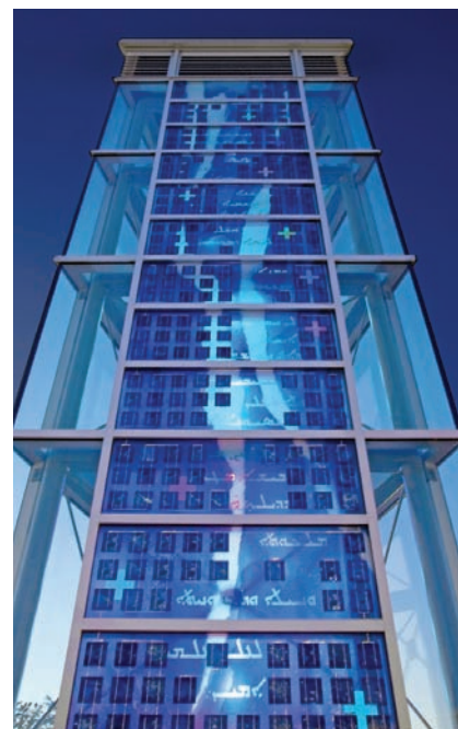
40-ft tower over Vancouver’s Regent College theological library combines art glass with solar power and LED lighting. Photo credit Michael Elkan.
